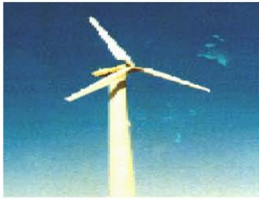
Wincon Danish WT, Stall regulated, Tubular tower, 100 KW
