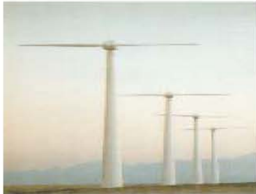
Ventis German WT, Pitch regulated Tubular tower, 2 blades, 100 KW
